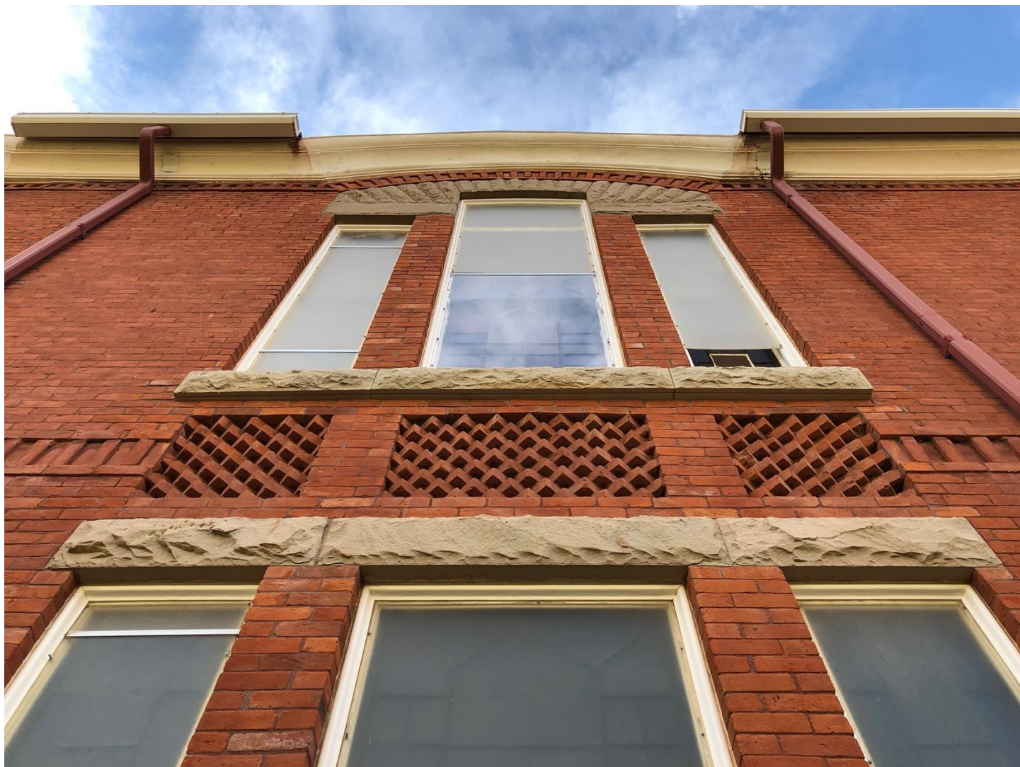
Photo 4 of 39. Temple Aaron, south side, detail of tripartite window arrangements, stone lintels and sills, decorative brick panels, and dentilated brick, view west-northwest.
